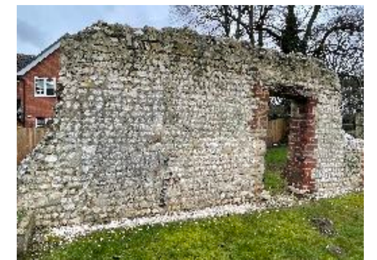
Clunch Stone Face loss following prolonged wetting and subsequent freeze thaw cycles.
